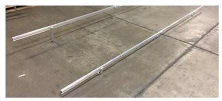
**COMPLETE ARRAY RAIL INSTALLATION: INSTALL SOLARMOUNT** RAIL ON BOTH SHORT AND TALL LEGS. CENTER RAIL LENGTH TO CREATE EQUAL CANTILEVERS FOR ARRAY. RAIL SPLICE(S) MAY BE REQUIRED TO ACHIEVE FULL ARRAY LENGTH.
