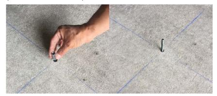
**INSTALL CONCRETE FASTENERS:** INSERT ANCHORS INTO HOLES AND SET PER MANUFACTURERS RECOMMENDATIONS. INSTALL ALL-THREAD TO APPROPRIATE DEPTH TO ALLOW FOR THICKNESS OF TILT LEG AND SERRATED FLANGE NUT.
