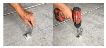
INSTALL TILT LEG: ALIGN HOLE IN SHORT TILT LEG WITH PROTRUDING ALL-THREAD AND SECURE WITH 3/8" SERRATED FLANGE NUT. TIGHTEN SERRATED FLANGE NUT TO TOROUE VALUE PROVIDED BY ANCHOR MANUFACTURER.
