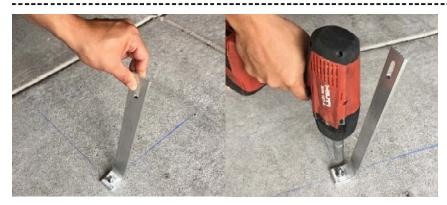
**INSTALL TILT LEG:** ALIGN HOLE IN LONG TILT LEG WITH PROTRUDING ALL-THREAD AND SECURE WITH 3/8" SERRATED FLANGE NUT. TIGHTEN SERRATED FLANGE NUT TO TORQUE VALUE PROVIDED BY ANCHOR MANUFACTURER.
