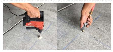
DRILL HOLES FOR CONCRETE ANCHORS: HOLE DEPTH AND DIAMETER SHALL BE PER CONCRETE ANCHOR/EPOXY MANUFACTURER. ASSURE ALL DUST AND DEBRIS ARE REMOVED FROM HOLES PRIOR TO ANCHOR INSTALLATION.
