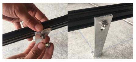
**INSTALL SOLARMOUNT RAIL ON TILT LEGS: UTILIZE TYPICAL** SOLARMOUNT 3/8" T-BOLT AND SERRATED FLANGE NUT TO FASTEN SOLARMOUNT RAIL TO SHORT AND TALL TILT LEGS. TOROUE 3/8 RAIL ATTACHMENT HARDWARE TO 30 FT-LBS.
